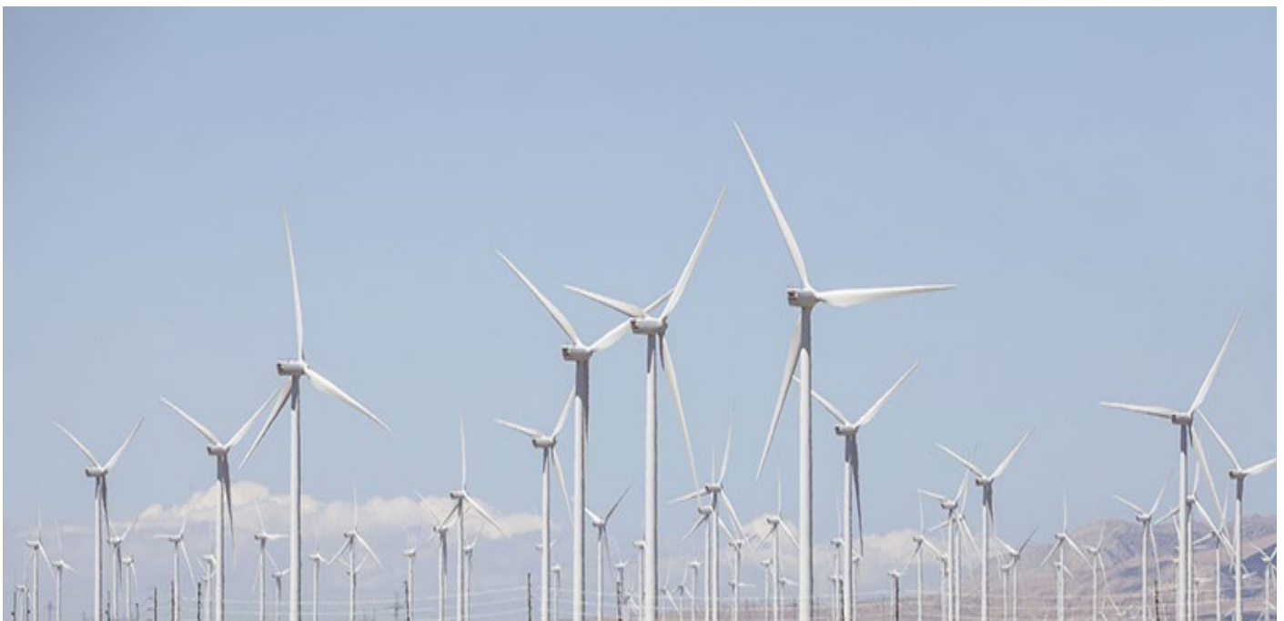
Figure 1: The De Aar Wind Power Project in South Africa (Source: Energy Capital & Power)
